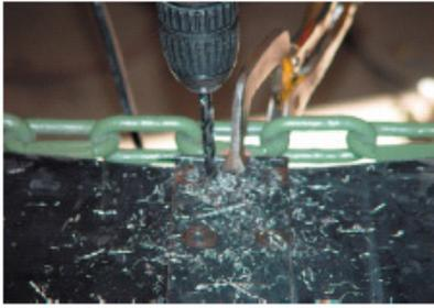
8. After pre-drilling all the holes on the top side of the feedbelt install the stainless steel tec screws and 1/4" washers.
